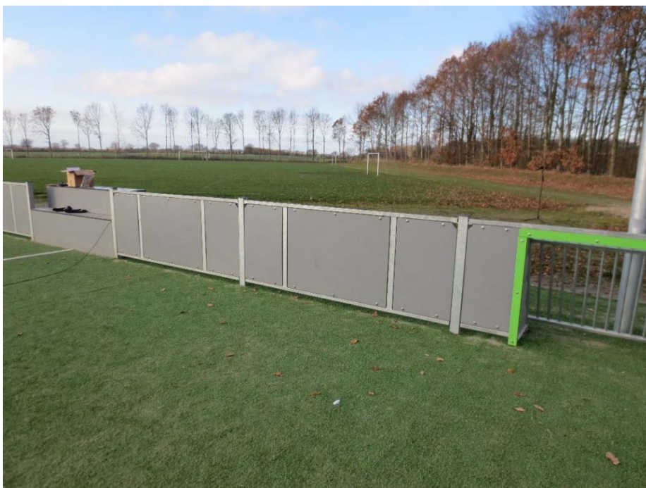
Figure 12 HDPE panel seen from inside the MUGA.
